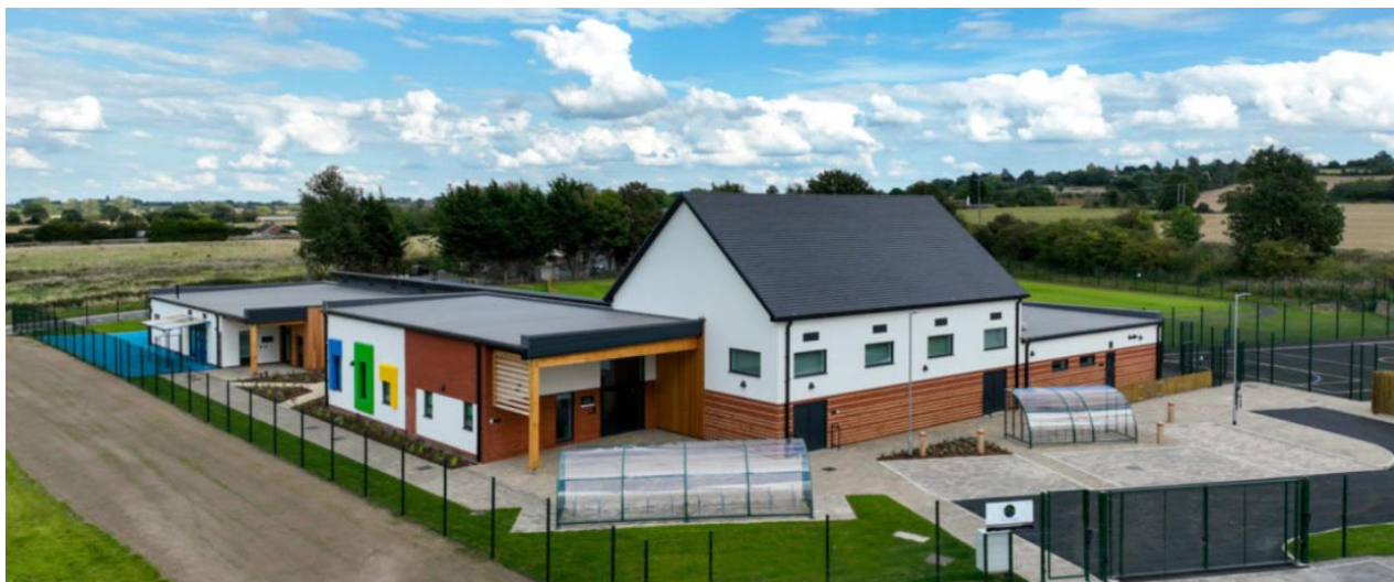
Figure 3: Newly constructed Allscott Meads Primary School by SJ Roberts Construction as a part of the TWC/2014/0113 Former British Sugar site, Allscott Opened September 2023
